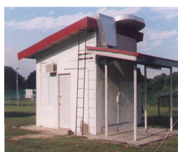
Fig. 16: Photograph of the solar dryer with V-groove solar collector
