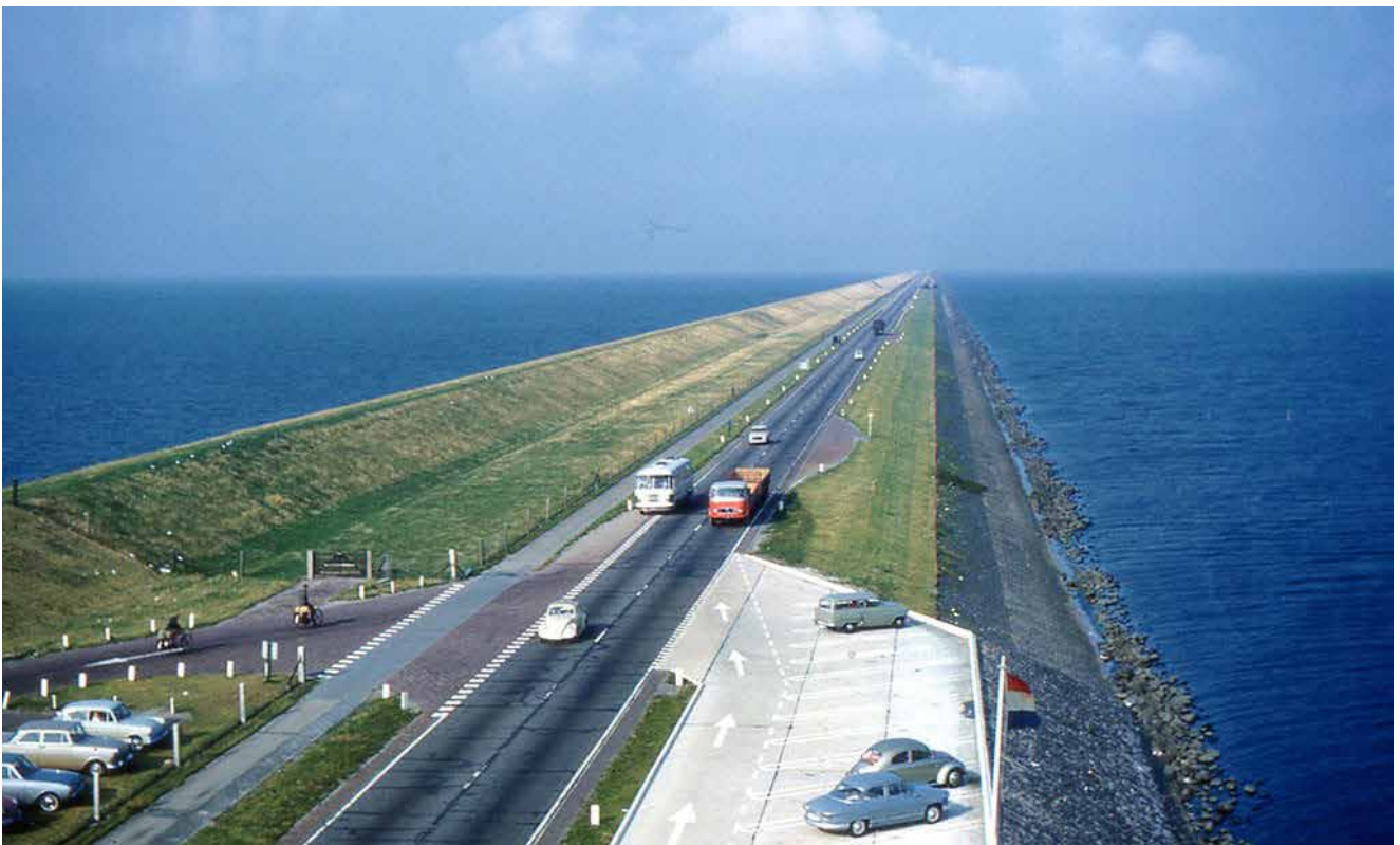
Figure 4: Levees in the Netherlands (Source: Waterisearth, 2016)
