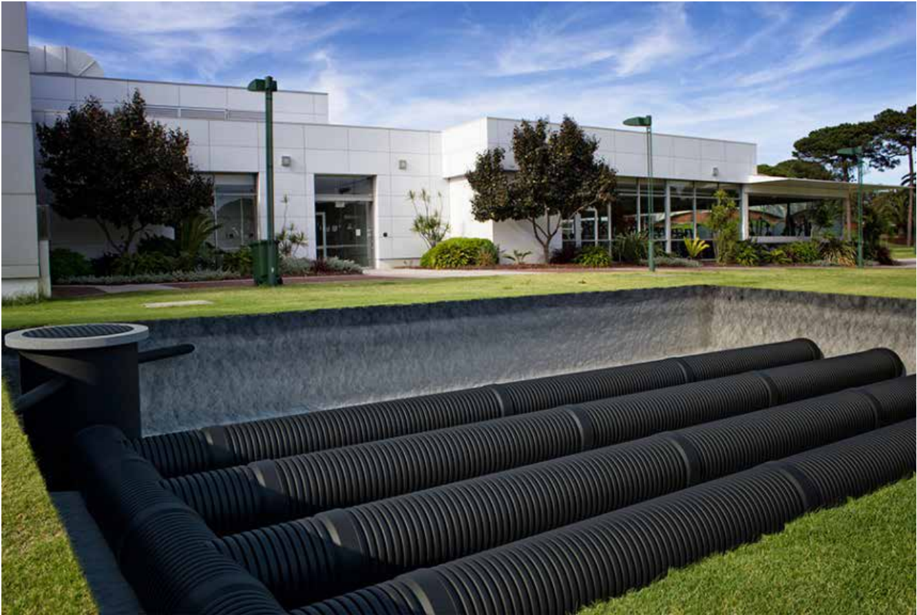
Figure 5: Stormwater Retention System in Australia (Source: Enviropipes2024)
