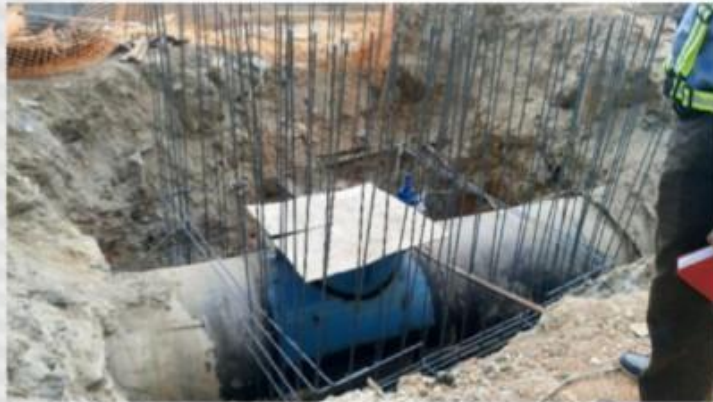
SYABAS sluice valve work on going.
