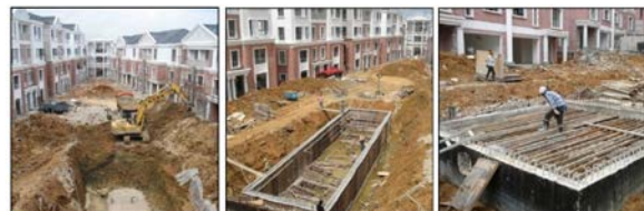
Fig. 4. Excavation, formwork, and casting the storage tank
