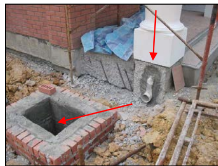
Fig. 3. The collection sump under construction
