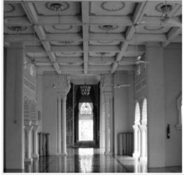
Figure 10.9 : Concrete ceiling with plaster finishes at the veranda area Source: IIUM, 2007
