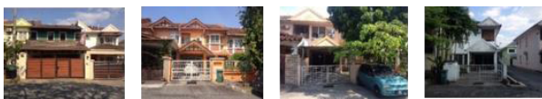
Figure 6: Types of front yard - from fully extended to original design (from left to right)
