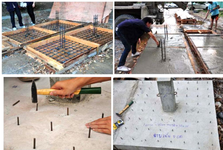
Figure 3 Preparation of test specimens
