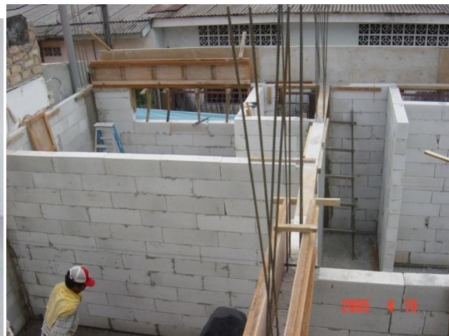
Figure 2: Lightweight Materials – here Combined Block with Polysterene (a) and full block Application in a Smart Cool Home ® (b)
