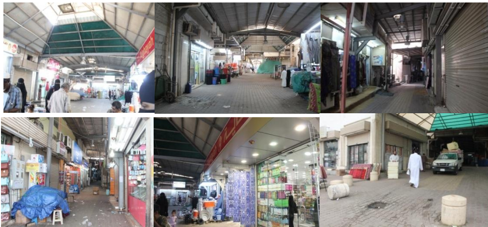
Figure (6) Shading the narrow alleys of the old souk with light steel elements, (Photos taken by the author in March 2015)
