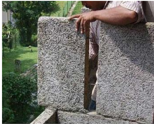
Figure 1: Wood-wool cemented wall construction board
