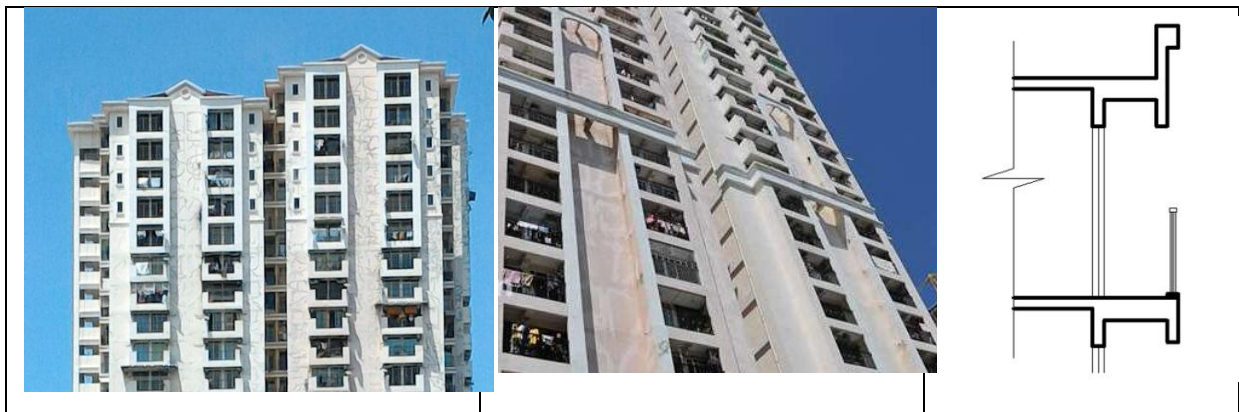
Figure 1. Halaman Kristal apartment with colonial architectural style (Left & Middle: Photos, Right: Section A-A)
