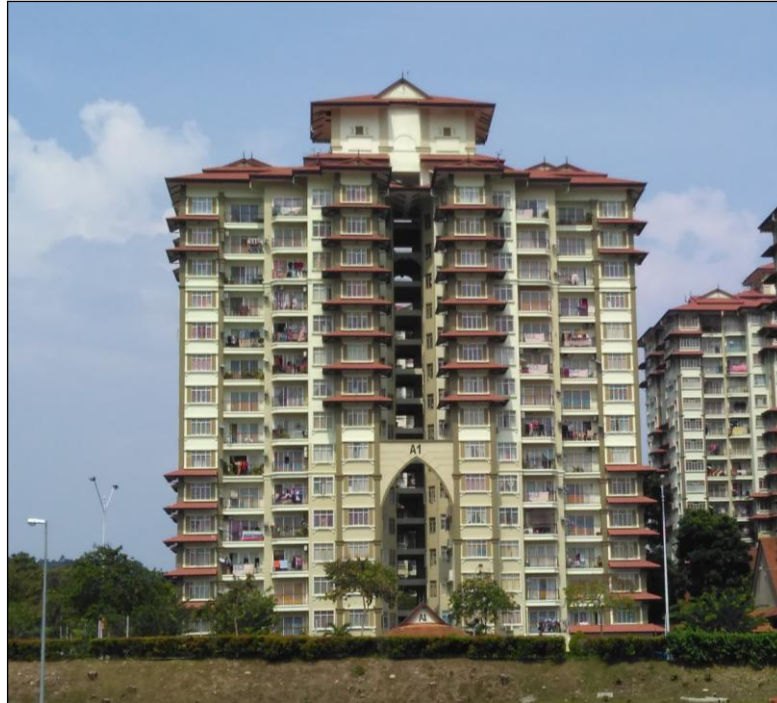
Figure 4. The first case study, vernacular style apartment.
