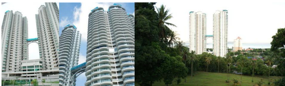
Figure 4: The View Building (Case Study) general views.
