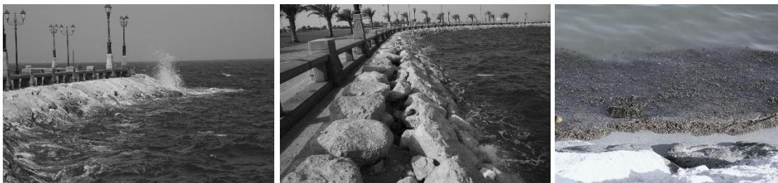
Figure 8: segment 3 affects by strong waves and tidal actions with severe disturbance of its elements and structures
