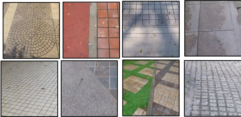
Figure 9: Existing types of ground surface materials used in KLCC area.
