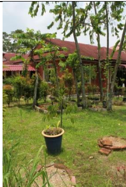
Improper placement of trees and lack of landscape maintenance lead to visual defects
