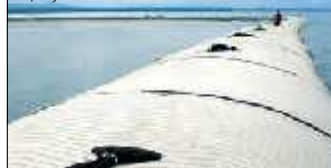
Geodyke in land reclamation, coastal protection and flood mitigation projects
