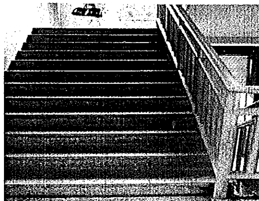
Figure 4. Consistent height of staircase riser (IBS Method)
