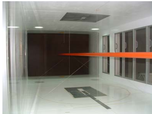
Fig. 1 Installation of static pipe in the wind tunnel.
