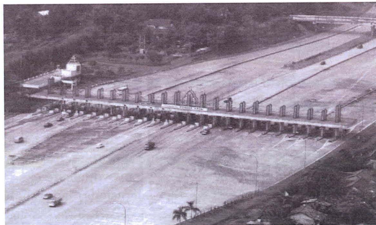
Fig. 14.1: A highway with a series of toll gates can be modeled by a simple queueing system.
