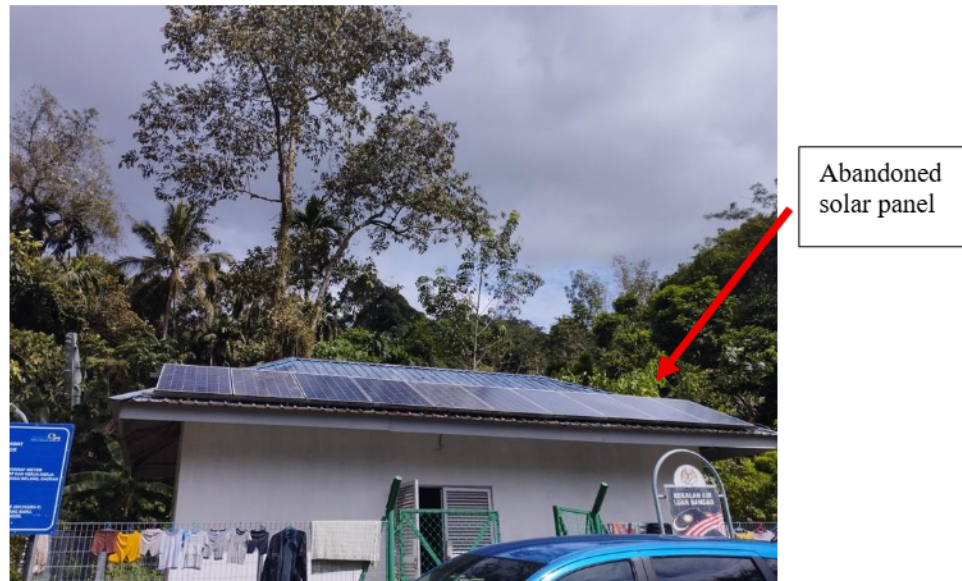
Figure 8. Abandoned solar panel assets from a previous solar electrification project at Kampung Sungai Relang (October, 2023).
