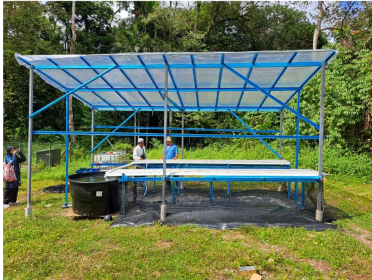
Figure 6. Installation of Aquagreen system at Kampung Sungai Relang (October, 2023).
