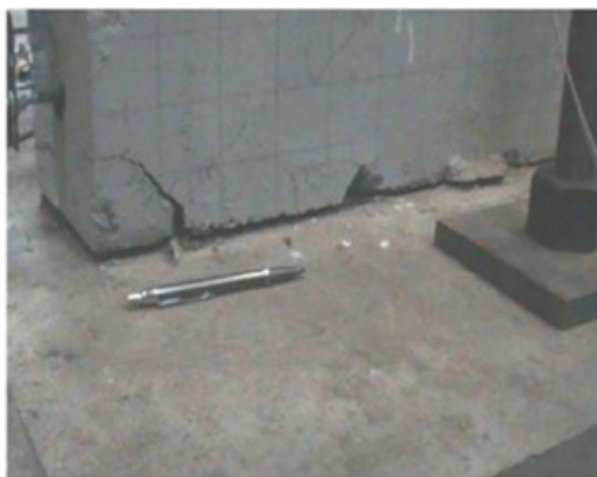
(a) Tie beam and foundation separation of experimental specimen (Triwiyono et al., 2020)
