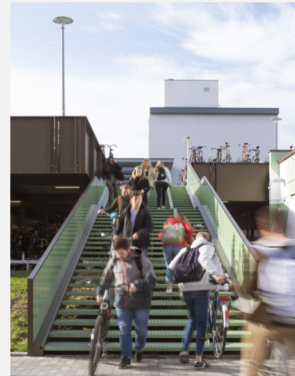
Figure 11: Staircase towards the second floor with bicycle railway
