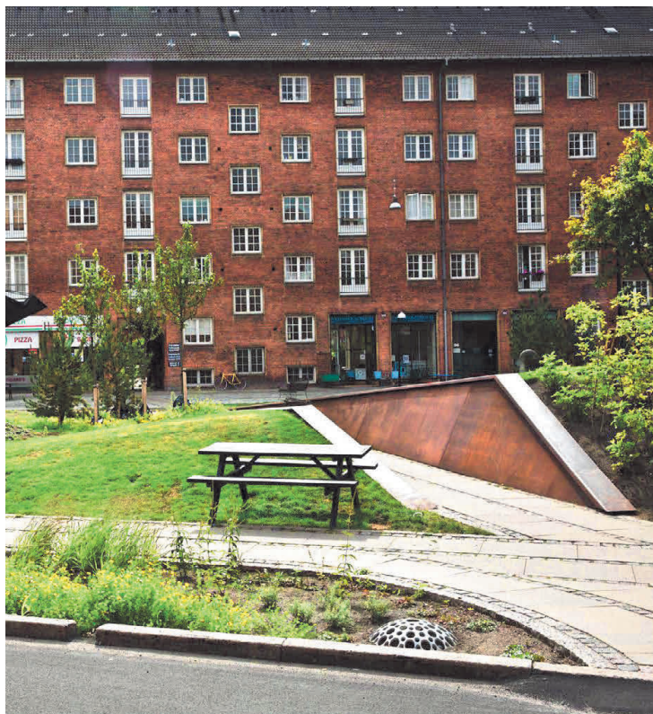
LEFT Tåsinge Square, Copenhagen, Denmark – this square garden was designed to collect and store rainwater in overcoming the frequent flooding at the basements of the neighbourhood premise. (Source: Publicspace.org)
