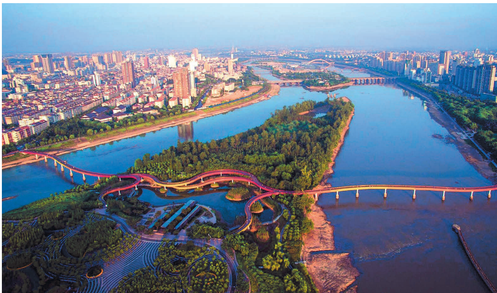
BELOW Yanweizhou Park, Jinhua City, Zhejiang Province, China – one of Kongjian Yu's iconic projects that was designed to curb annual flooding due to Jinhua's monsoon climate. (Source: landscapearchitecturebuilt.com)
