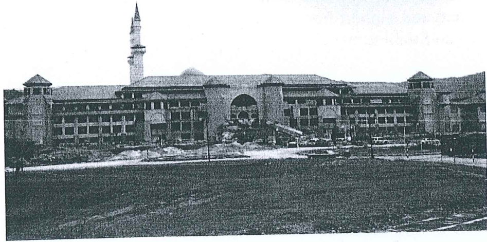
IIUM Gombak campus under construction
