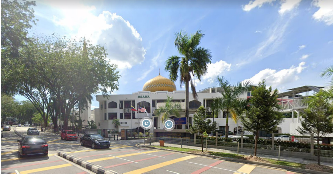
Fig. 3. Masjid Saidina Abu Bakar As-Siddiq, Bangsar: Emphasis on functionality to adopt the traditional Malay house as precedence. (Source: Google street view)
