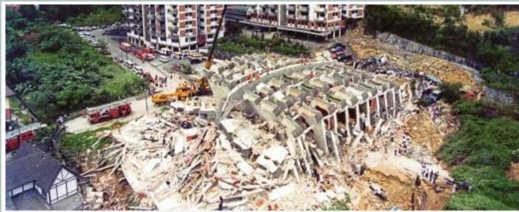
The collapsed Highland Towers condominium in Ulu Kelang, Selangor. Picture by Kamarudin Ahmad https://www.nst.com.my/news/2015/09/remembering-highland-towers-tragedy
